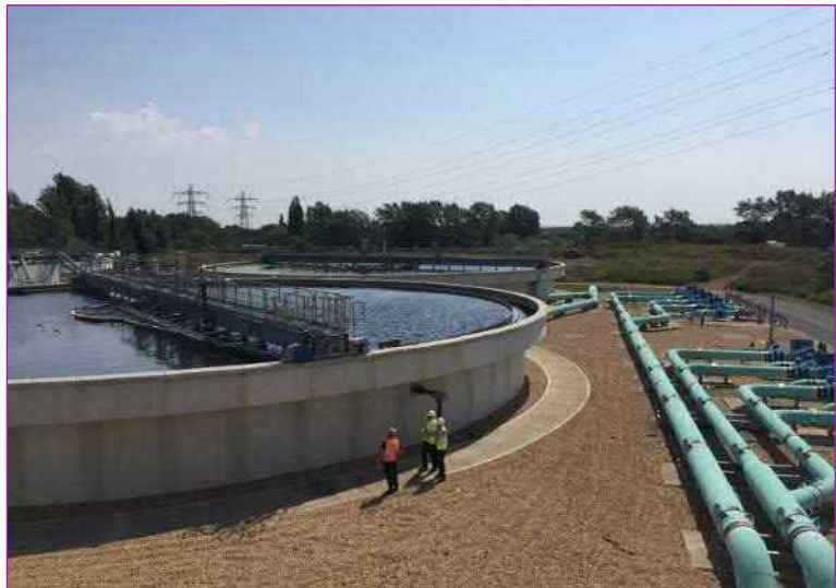
Figure 2-9: Existing Cambridge Final Settlement Tanks
