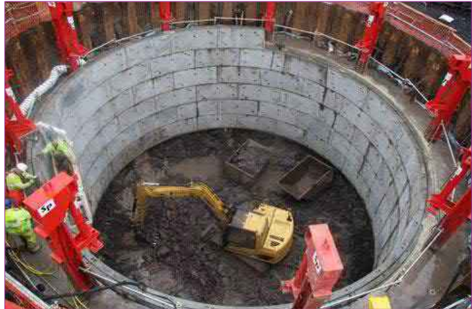
Figure 2-5: Example shaft construction
