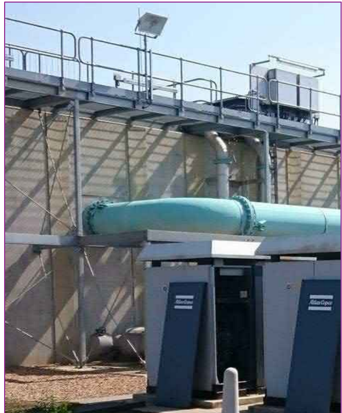
Figure 2-19: Example task lighting
