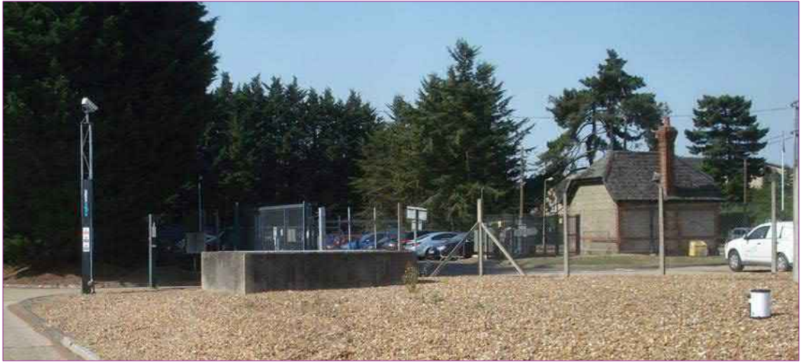
Figure 2-18: Example fencing and CCTV camera
