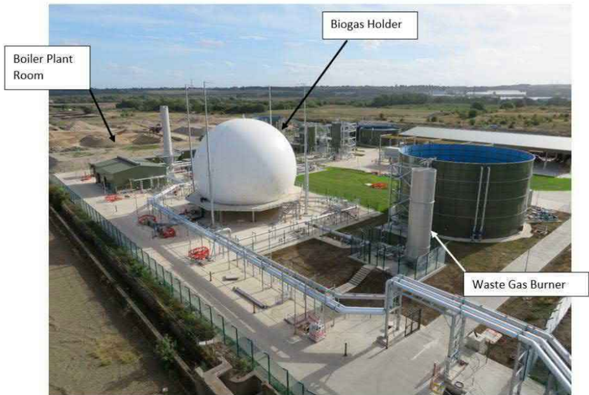
Figure 2-16: Knostrop sludge treatment centre
